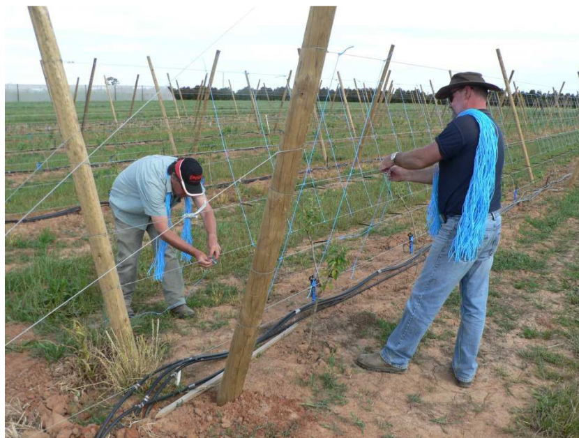
Figure 2: Installing 50cm guiding strings
