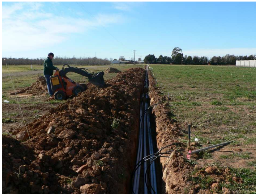
Figure 1: Installing irrigation
